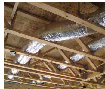
Ducts are run straight and supported properly.
